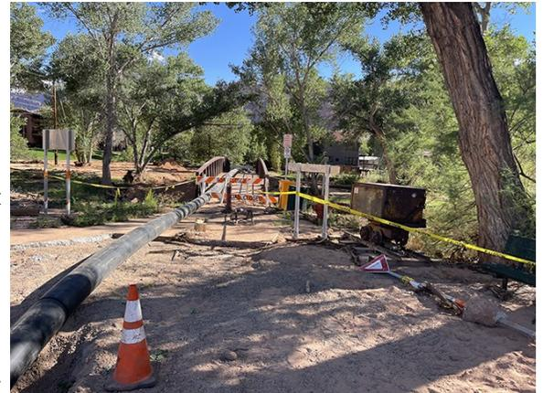
This temporary main water line was installed in September after the line running under Mill Creek was destroyed during the flood on Aug. 20, 2022.
